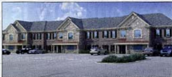
Three new office-condominium units are under construction at 5080 Wooster Pike, across from Amideer Park in the Linwood area. The long standing C.P.A. firm of Ernst and Rabe will be moving their operation to the new location in early fall.
